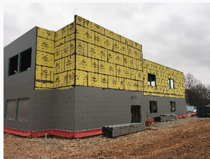
Exterior Sheathing, Air Barrier, & Brick Clips
