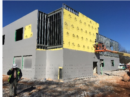
Exterior Sheathing, Air Barrier, & Brick Clips
